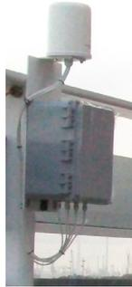
Outdoor MIMO Omnidirectional Antenna Installed With The 12" x 10" x 6" Polycarbonate Enclosure
